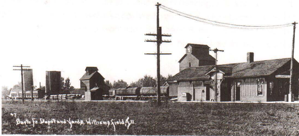
The Farmers Elevator and Railroad switching yards
